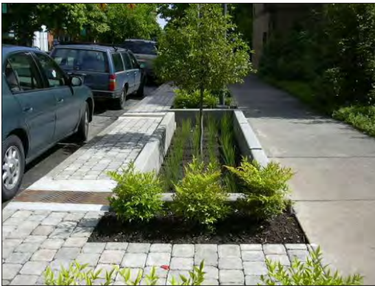
Rain gardens between sidewalk and parking lane drain stormwater runoff and provide space for vegetation.
