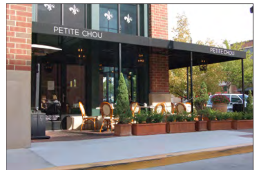
Canopy protects outdoor seating area.
