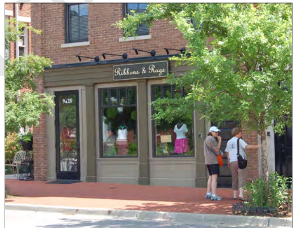
Suitable facade transparency at the pedestrian-level.
